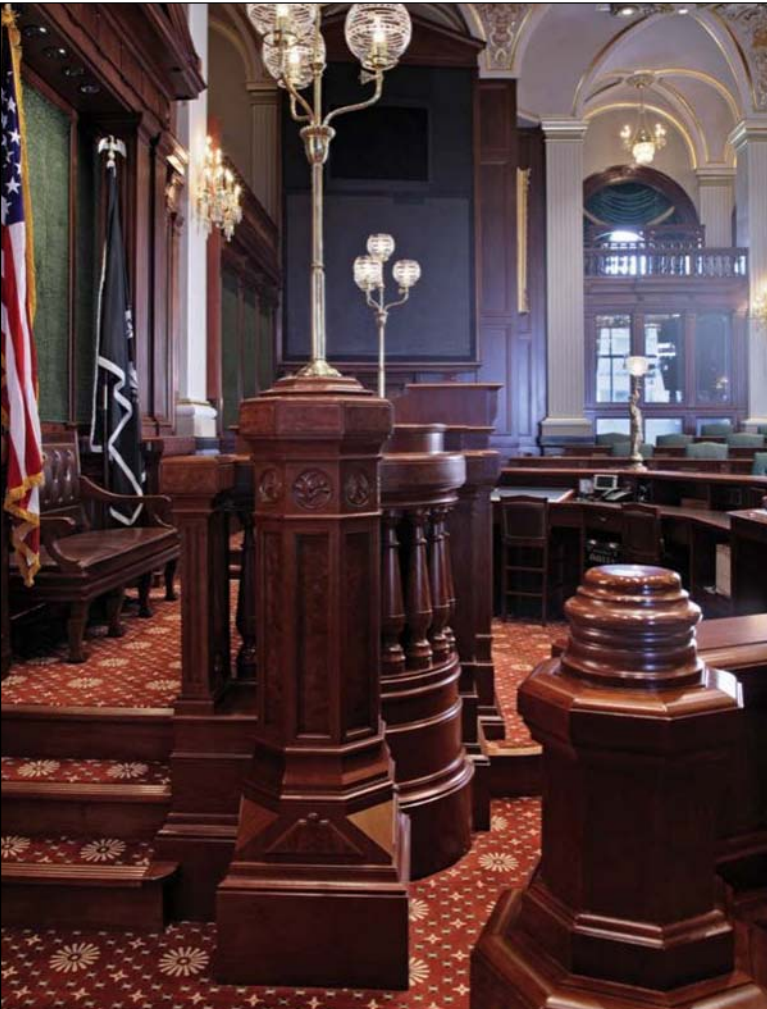
▲ AT THE ENTRY PORTAL, original hand-carved decorative panels were refinished and reinstalled in new wood surrounds based on photographs of the original work. ▼ Elaborate wood bases were constructed to accommodate decorative lights, below.
