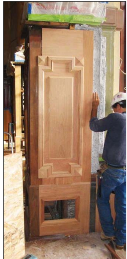
▲ MATCHING AND INSTALLING the new wood surrounds.
