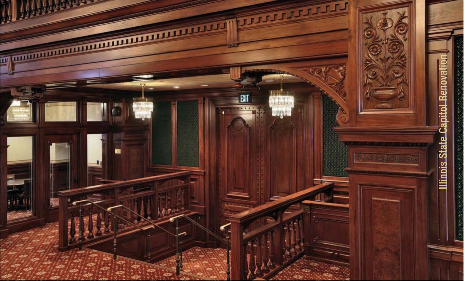
▲ AT THE ENTRY PORTAL, original hand-carved decorative panels were refinished and reinstalled in new wood surrounds based on photographs of the original work. ▼ Elaborate wood bases were constructed to accommodate decorative lights, below.
